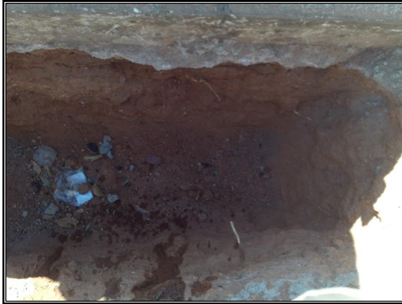
Plate 6: Subgrade material encountered in IP4
